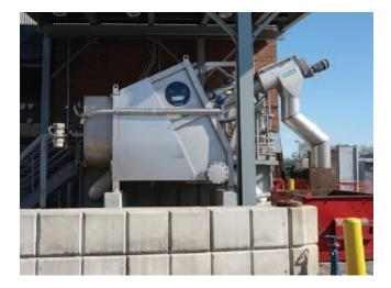
A heat exchanger using incinerator scrubber water allowed for a low cost hot water spray system. This has provided an added side benefit and has assisted in the overall maintenance efficiency for the BEAST.
